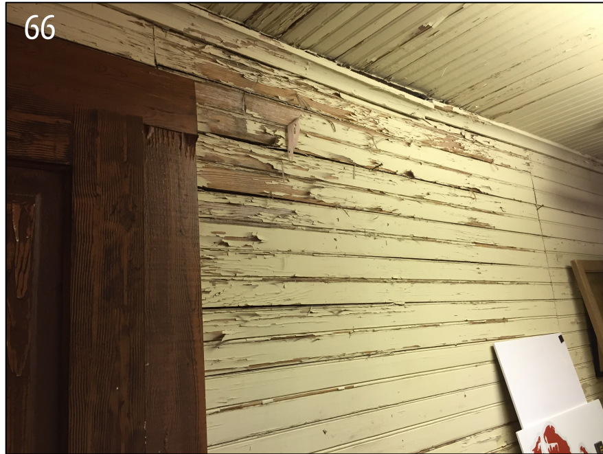
Figure 29. Moisture damage in room 219, instance 66.
