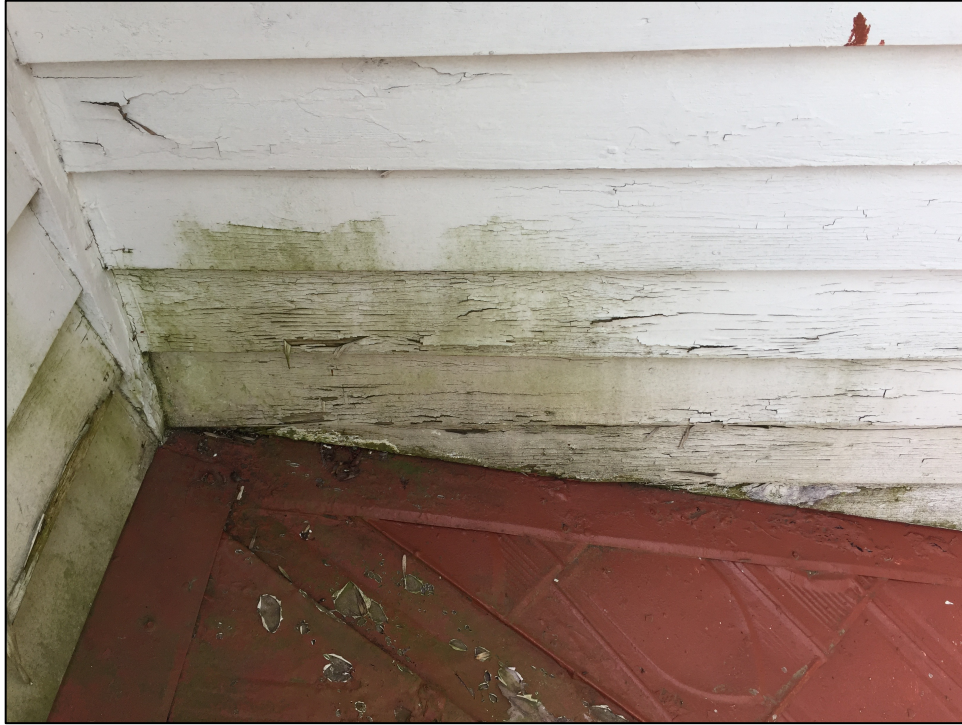
Figure 35. Moisture damage on the lower siding boards above the second floor roof.
