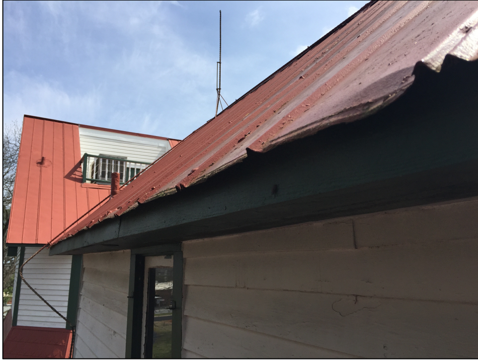
Figure 33. The upper roof has no gutter or drip edge.
