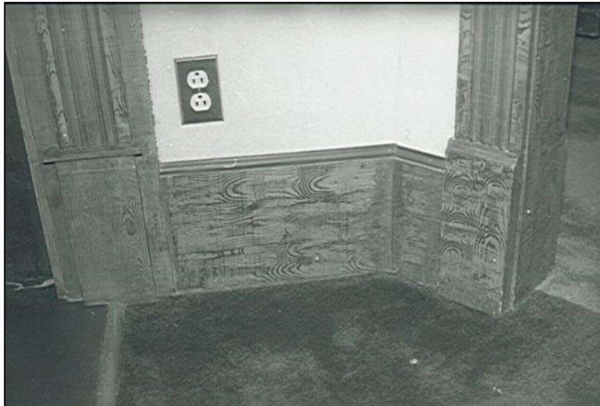
Figure 22. Photograph from early 1980s of baseboard, base of doorframe, and base of fireplace in gallery room 216 (scanned copy of photograph from the North Carolina Preservation Office's file on Lucas Mansion).
