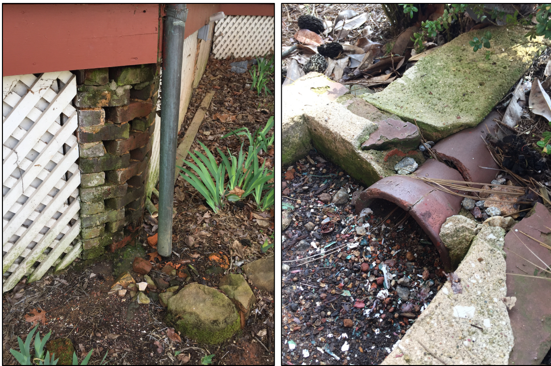
Figure 38. Compromised water drainage from down spouts.
