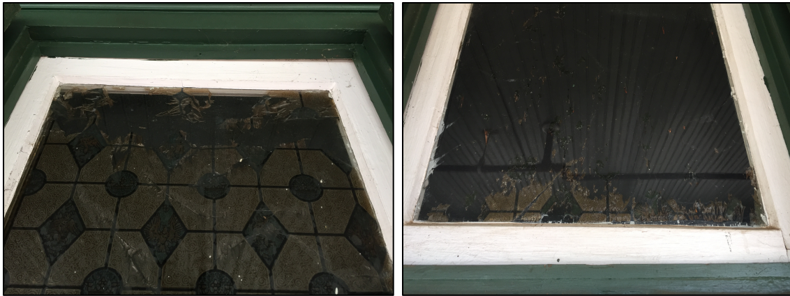
Figure 24. Windows on the west wall room 216 that have a decorative film that has deteriorated.
