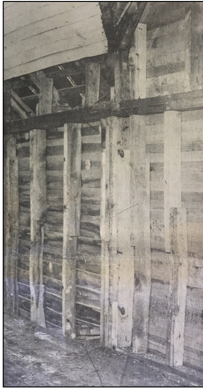
Figure 40. Photograph of 3 rd floor wall striped down to the stud (Joines, 1982).
