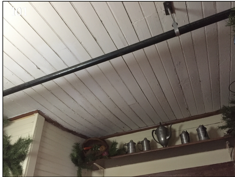
Figure 32. Sag in the ceiling of the historic kitchen (room 111) that continues to progress; instance 101.
