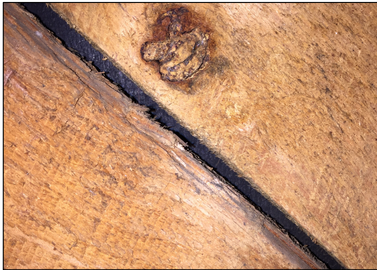
Figure 8. Thin layer of black paper-like material found between siding and sheathing. 11
