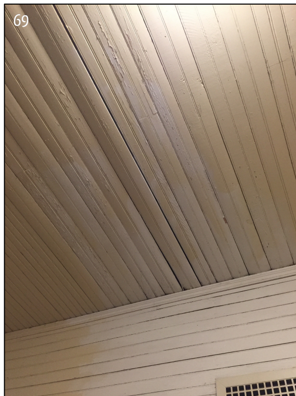
Figure 30. Moisture damage on the ceiling of room 219, instance 69.
