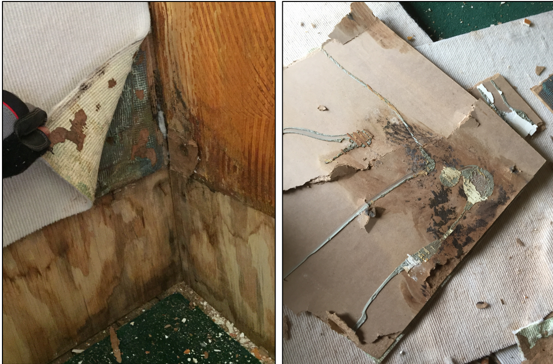
Figure 41. Molding and water stained material from northwest corner of room 217
