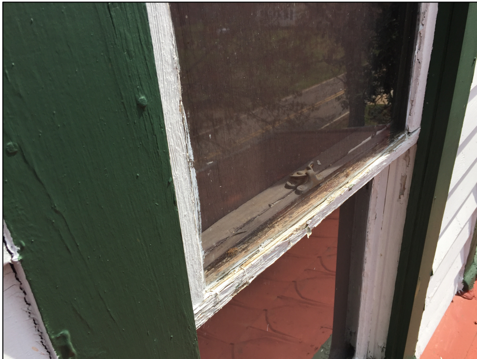
Figure 34. Third floor window with considerable moisture damage.
