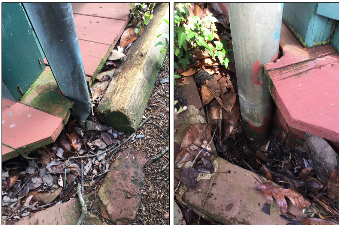
Figure 37. Compromised downspouts on the west side of the building.
