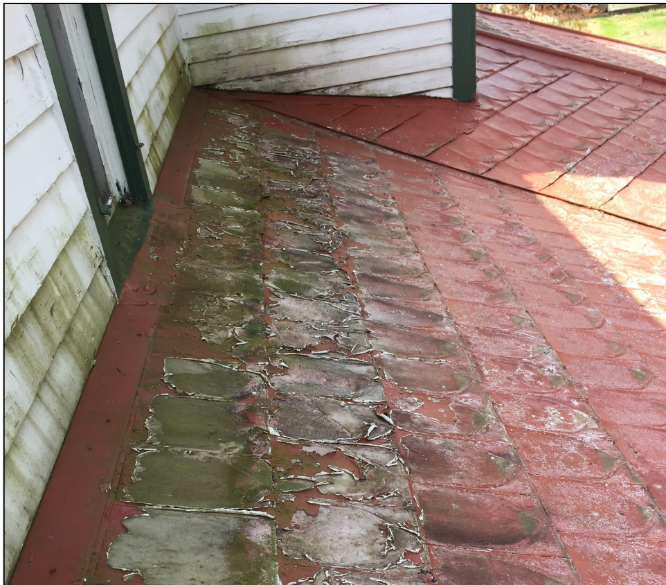
Figure 36. Peeling paint and moisture damaged siding on the second floor roof.
